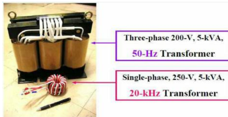
Fig. 4. Comparison of conventional and highfrequency transformer
